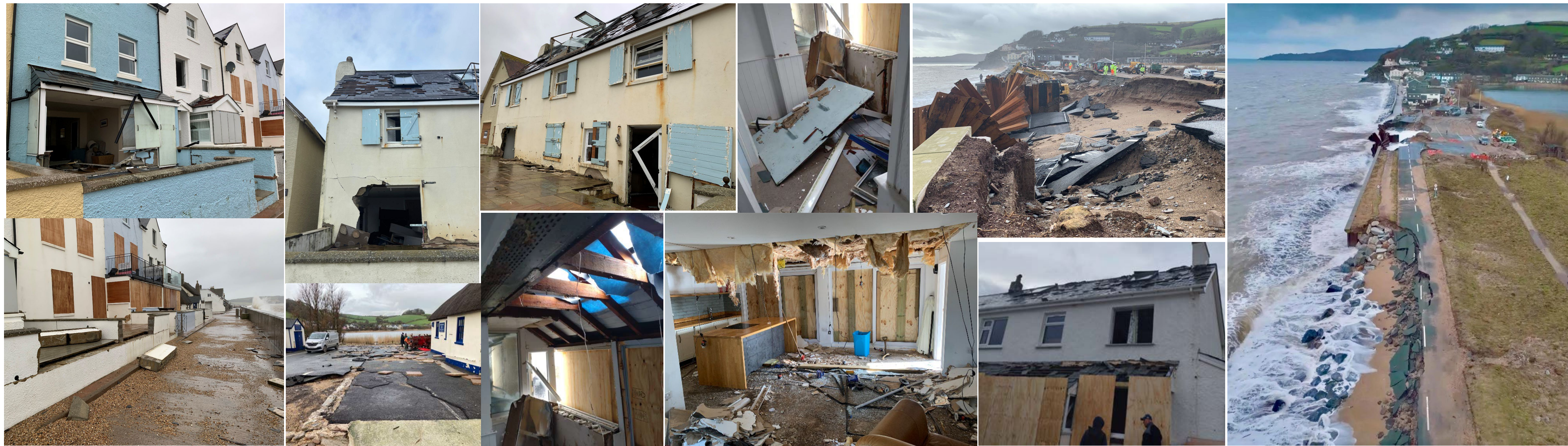
Fig 4. Between Christmas Day and mid March, Start Bay experienced 12 'storm' events, with the most devastating being on 24 th January (Storm Ingrid) and on the 3 rd /4 th February. These caused devastating damage to the frontage properties, very significant trauma for local residents and property owners, and the catastrophic breaches to the A379.
