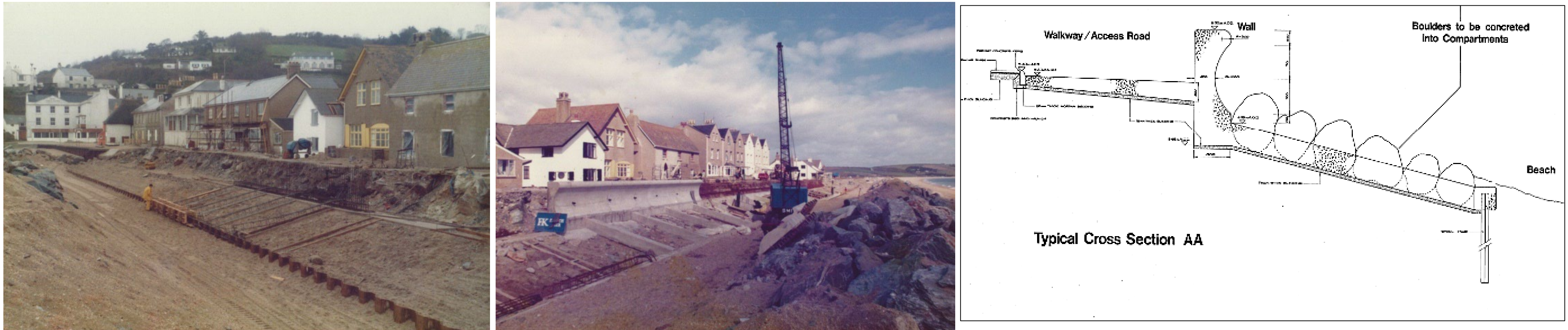
Fig 2. The Sea Defences consist of a reinforced concrete curved sea wall, with a sloping concrete/rock revetment, and 6m long toe piles (above). The reinforced concrete sea-wall, road-way behind it and the revetment's beams are all structurally connected together. Beach levels were envisaged to fluctuate, broadly between the top and bottom of the revetment.
