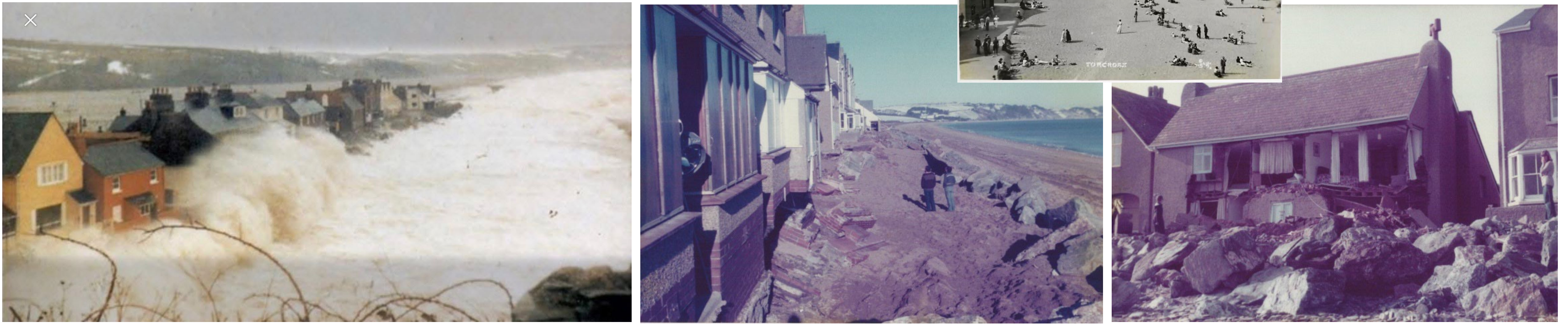
Fig 1. Historically Torcross predominantly relied on its large shingle beach for storm protection, however severe storms in 1978/79 caused huge damage to the village (above), and resulted in the current Torcross Sea Defences being constructed by the then South West Water Authority in 1980.
